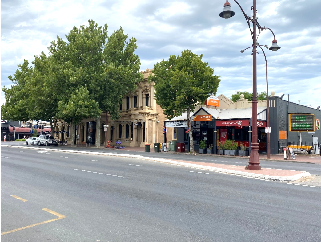
Figure 3.5 – western side of O'Connell Street opposite subject site
