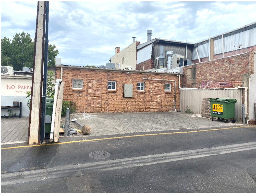
Figure 3.2 – rear of subject site viewed from Lohrman Street
